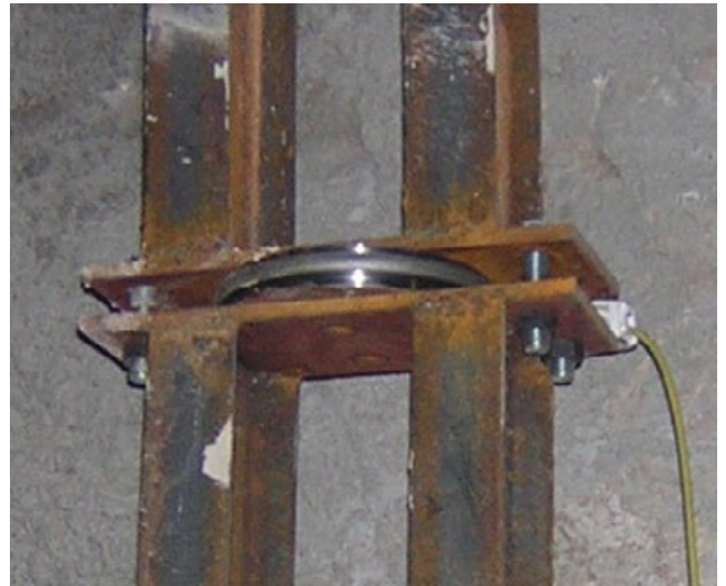
Load cell between two steel lining sections
